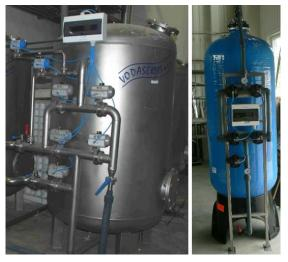
automatically in time or after passing a determined amount of water through the pulse inlet water meter. At the time of washing and filter regeneration, the water is not regulated. Regeneration salt tablets are used for regeneration. The salt consumption is 0.2 kg/l of ion exchange cartridge.
